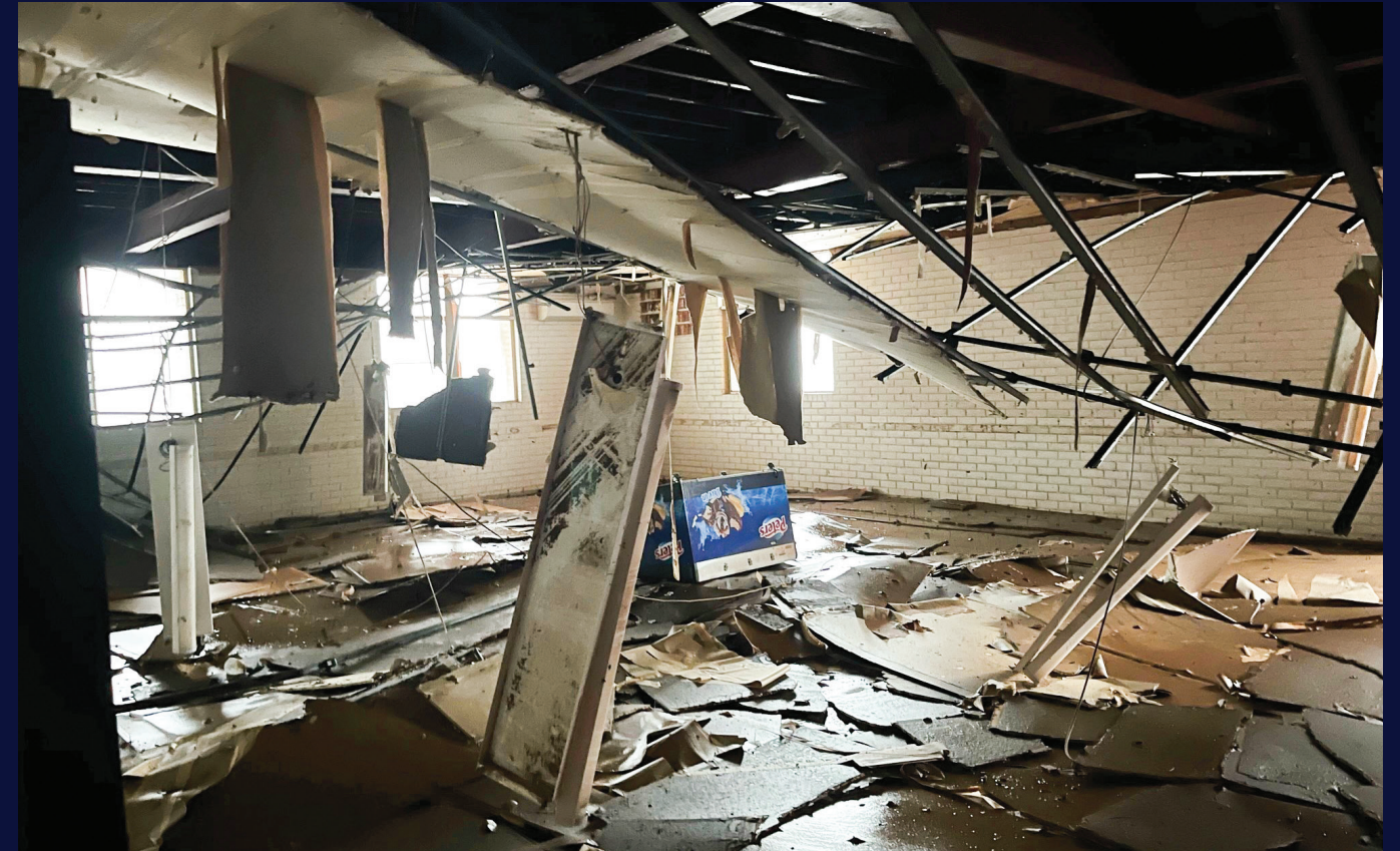
Lismore ground floor ceiling collapse 6 March 2022.
